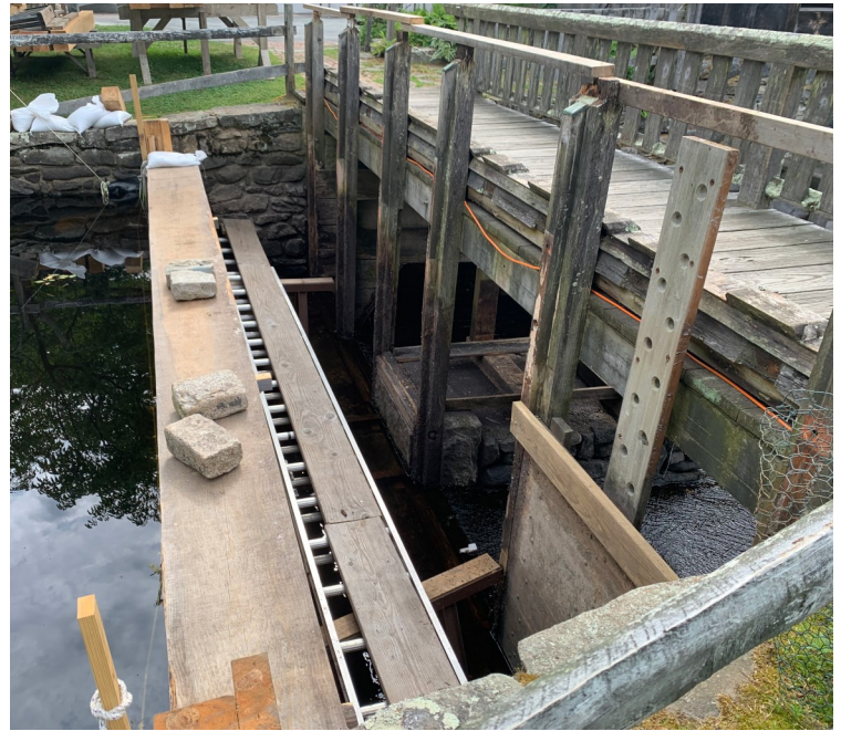
View into the coffer dam, and through the removed gates
