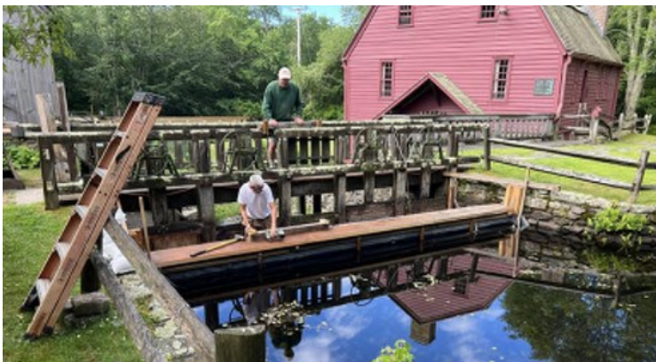
Shrake Millwrights at work on the construction of the coffer dam
